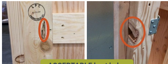
ACCEPTABLE knot holes
